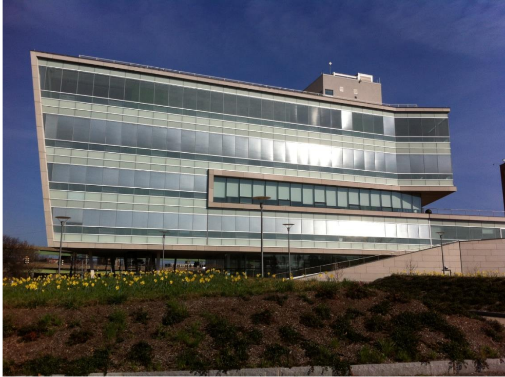
Figure 3.31 South façade of Syracuse CoE Headquarters building
