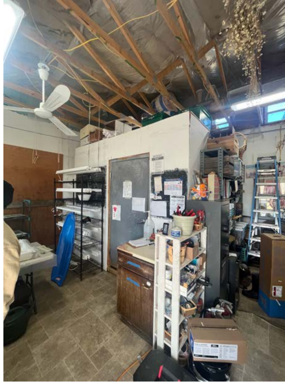
Figure 1.03 - Existing building on farm site taken on Feb 13, 2024
