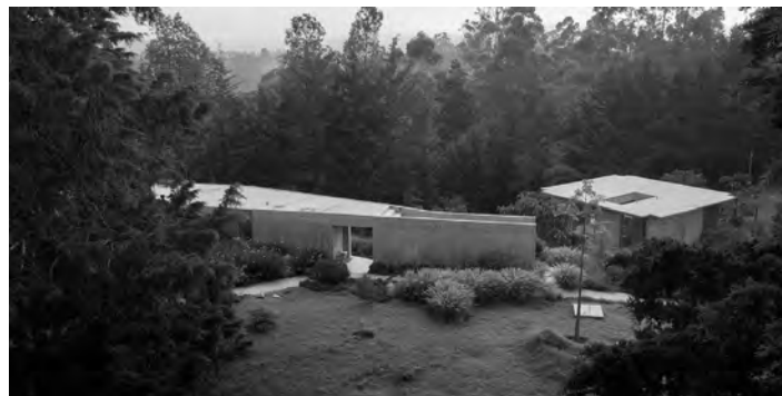
Ballen House | © LCLA OFFICE
