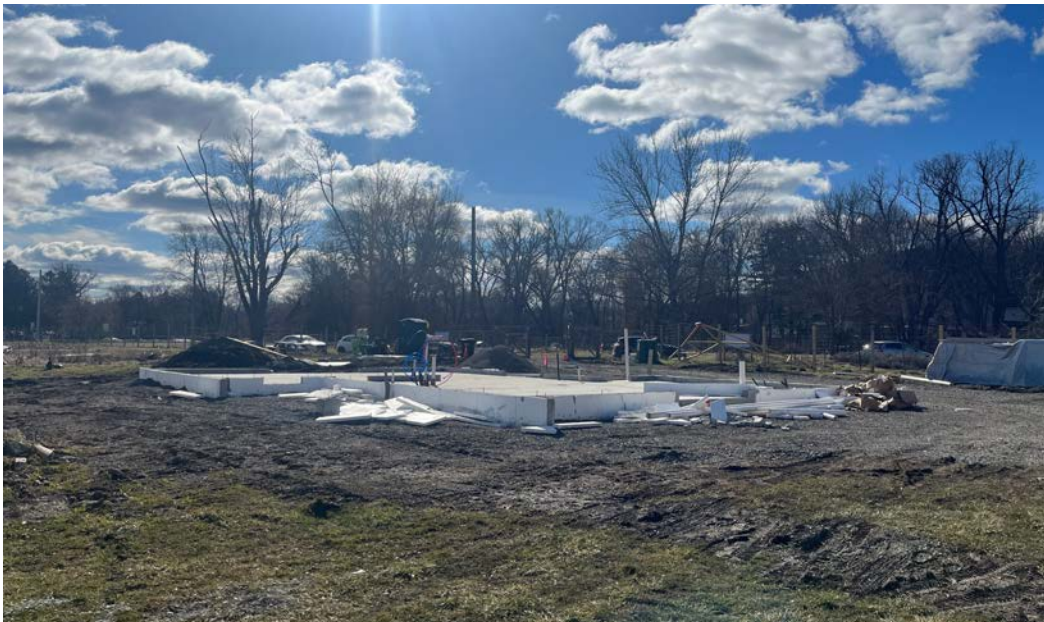
Figure 1.02 - Construction progress on Brady Farm new building as of Feb 13, 2024
