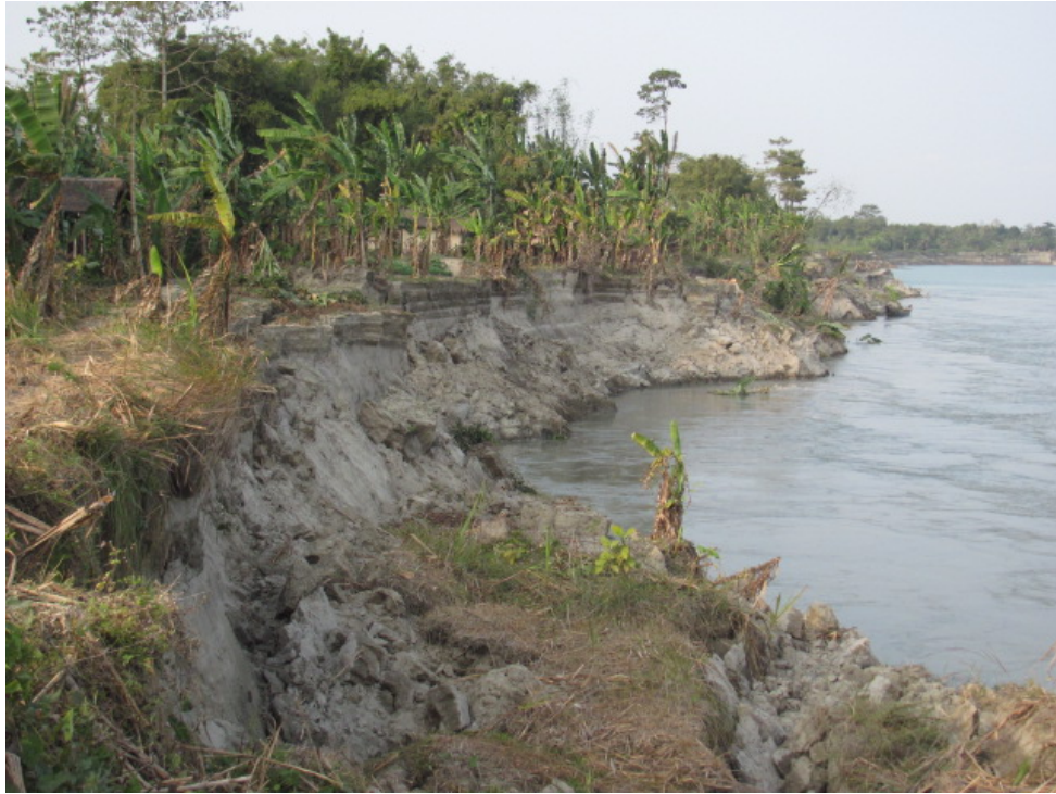
Figure 14: Riverbank erosion. Salmora, Majuli, December 2012.
