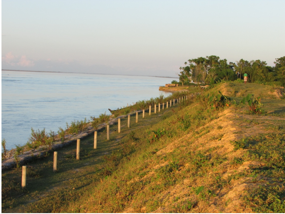
Figure 16: Earthen embankments at Rohmorja. September 2013.
