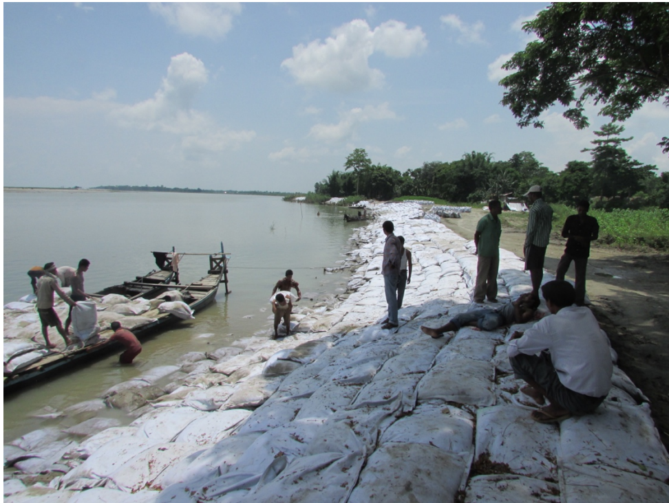
Figure 15: Sandbags as flood protection measure. June 2013.
