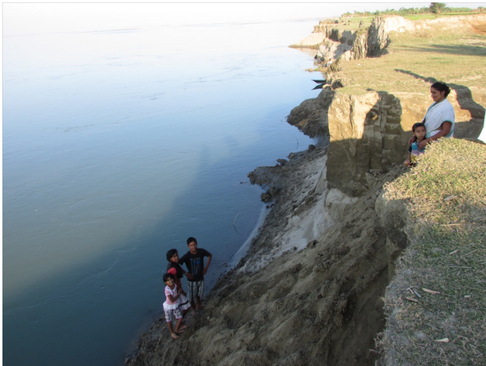
Figure 13: Riverbank erosion. Lahorighat, October 2013.
