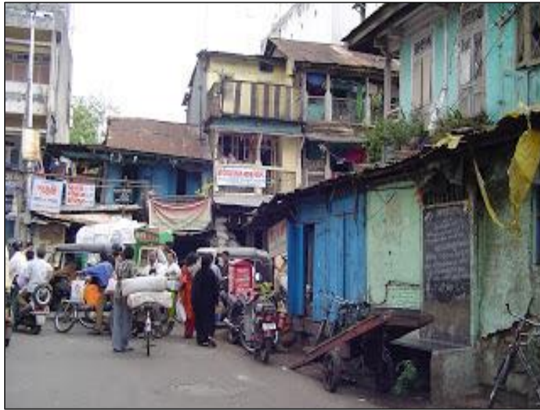
Photo 1.5: The "unruly" spaces of eastern peths in Pune. Most of the lanes are narrow and choked with traffic. The houses, as can be seen in the image on the right, are old and crumbling.
