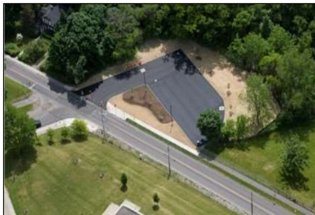
Figure 20: Hughes Magnet School parking lot permeable pavement
