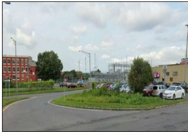
Figure 12: City parking lot 4 rain garden
