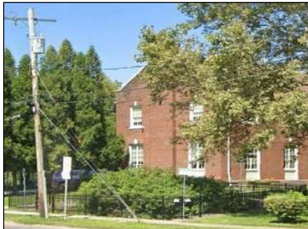
Figure 14: White library infiltration trench
