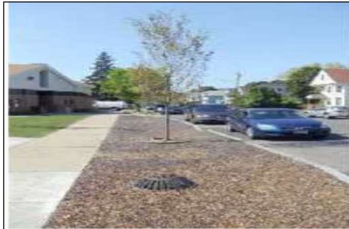
Figure 16: Mundy library infiltration trench
