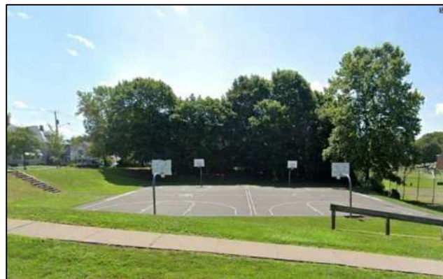
Figure 18: Lewis Basketball Court permeable pavement
