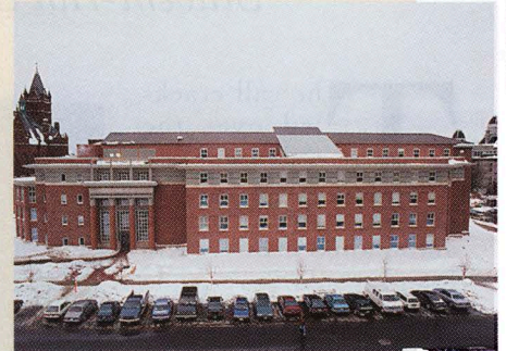
SU's newest structure, Melvin A. Eggers Hall, is home for the Maxwell School.
