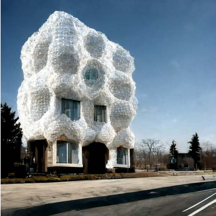
A building that has the texture of and looks like bubble wrap
