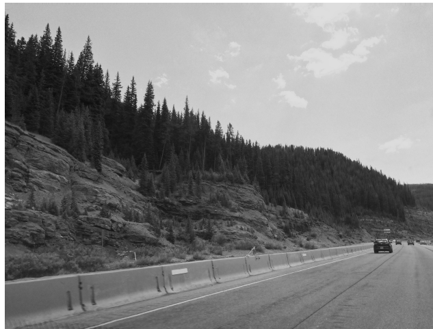
Figure 4.1. Rock cuts mimic naturally existing faces, facilitating the principle of vision in motion , west side of Vail Pass. Photo by author.
