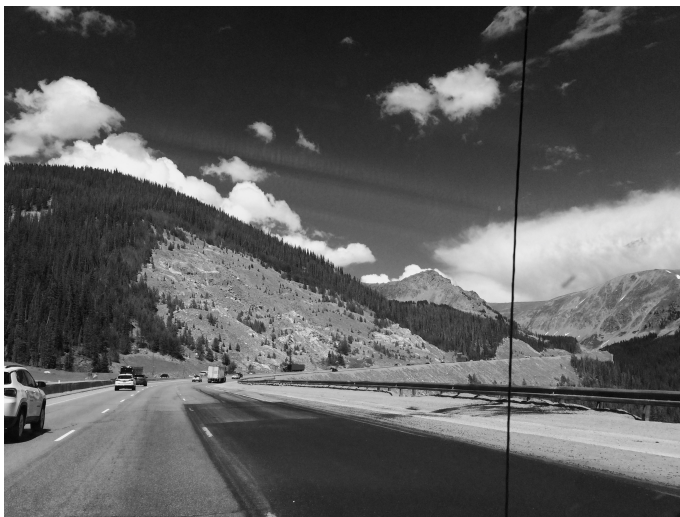
Figure 2.2. Eroded hillsides, west side of Eisenhower Tunnel. Photo by author.
