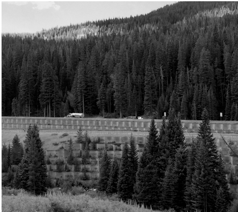
Figure 4.3. Custom barrier walls create unified design language throughout the drive, west side of Vail Pass. Photo by author.
