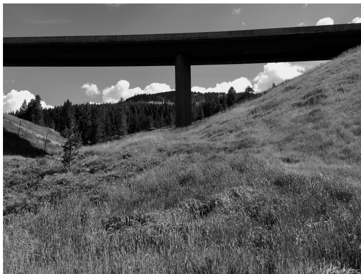
Figure 1.3. Bridge as seen from bike path, east side of Vail Pass. Photo by author.
