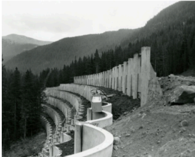
Figure 3.3. Interlocking retaining walls minimize visual massiveness. 163
