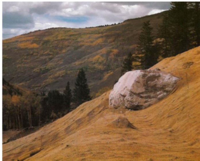
Figure 3.2. Rocks were placed on disturbed slopes in a naturally appearing manner. 162
