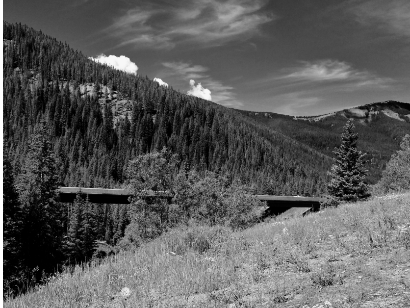
Figure 3.4. Bridge anchored into hillside reduces need for support columns, west side of Vail Pass. Photo by author.
