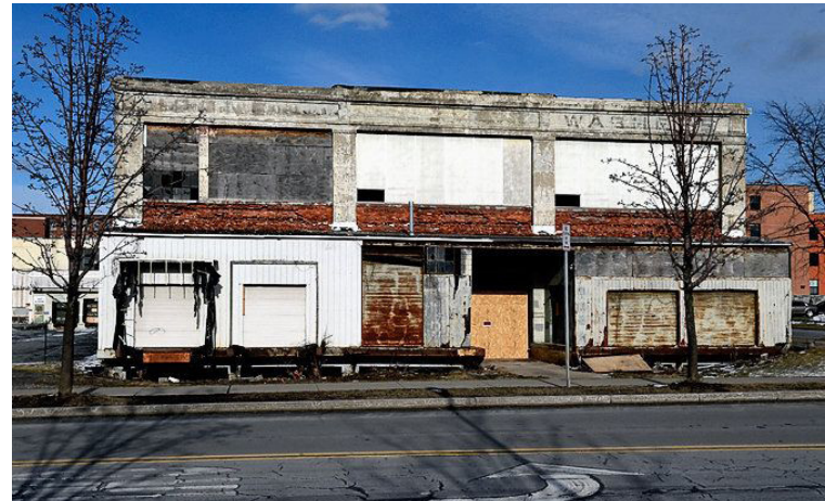
the Easy Washing Machine factory building, Solar and Spencer St.
