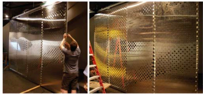
4.1.7 Full-scale working prototype of Eclipsis screen design with rotated tabs
