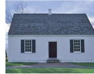
Vernacular typology, Cape House New England, USA c. 1980
