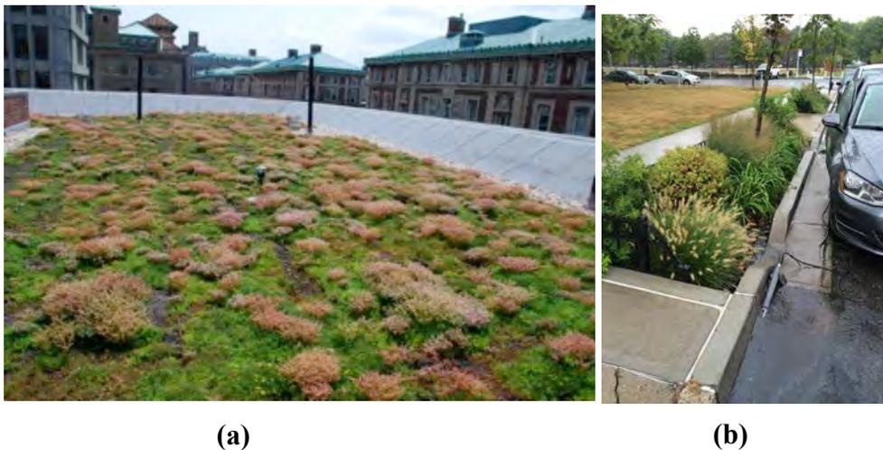
**Figure 3.** a) Green roof on a Columbia University building, and b) Right-of-way bioswale in the Bronx, New York City. Image (a) courtesy of Stuart Gaffin, Columbia University. Image (b) courtesy of Nandan Shetty, Columbia University.
