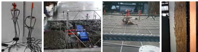
Figure 3. Installation of T-H sensors
