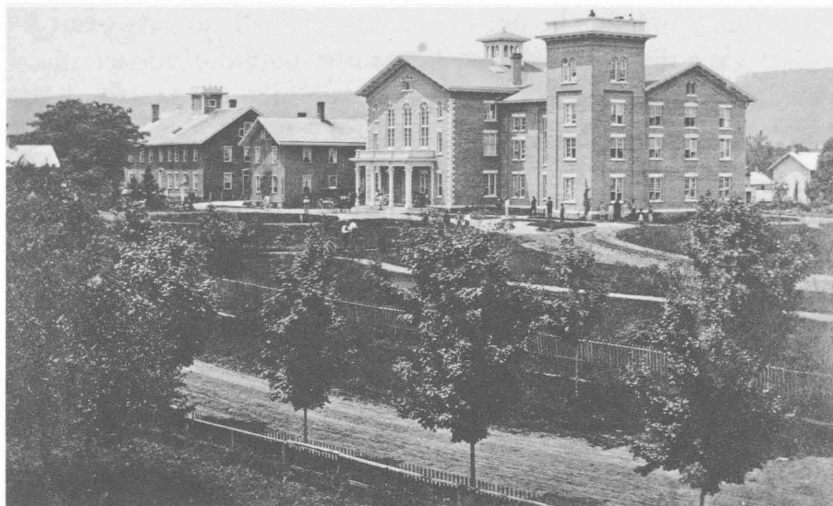
Fig. 4. A June 1863 photograph showing the New Mansion, the first Children's House, and the Old Mansion.
