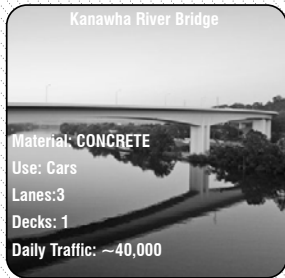
Kanawha River Bridge
