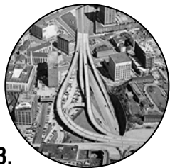
3. Fig 6.2 Boulevard of the Allies and Crosstown Boulevard Intersection
