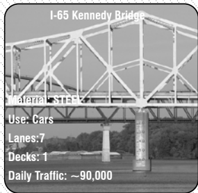
I-65 Kennedy Bridge
