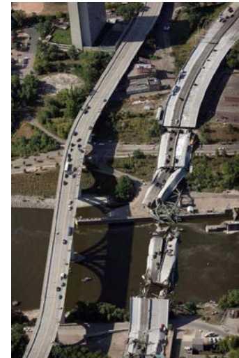
Fig 3.0 I-35W Mississippi River bridge
