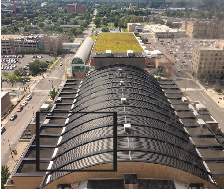
Figure 3.1: Aerial view of traditional roof on War Memorial building in downtown Syracuse, NY. The area of the roof that drains to the sampling pipes is indicated in the black box. This area is 1176 m 2 , measured using CAD by Onondaga County staff.
