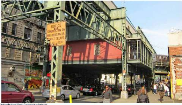
Nassau Street Station
