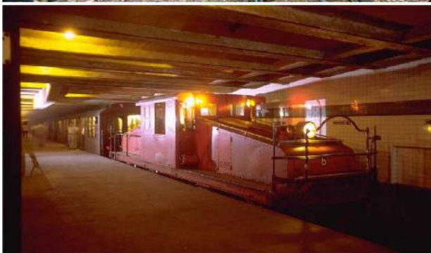
Court Street Station
