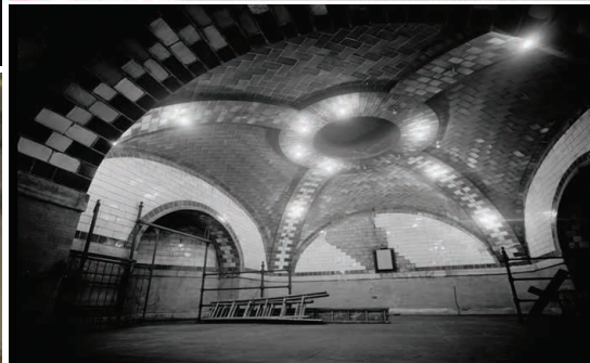
City Hall Station
