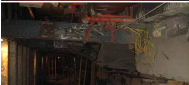
8th Street Avenue
