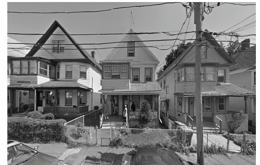
ATLANTIC STREET HOUSING UNIT Land Use: Three Family Housing Unit Year Built : 1910
