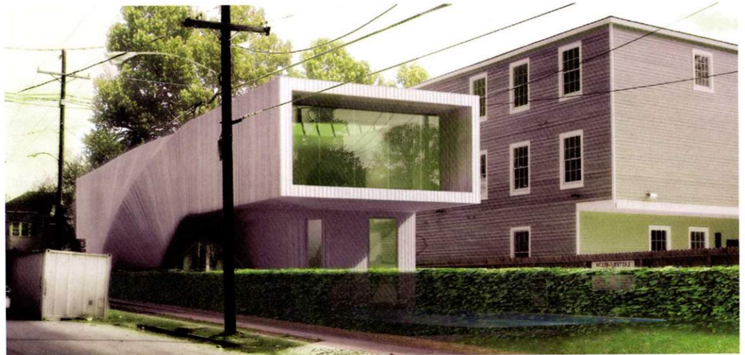
Ammar Eloueini Digit-ALL Studio; J-House , New Orleans, under construction
