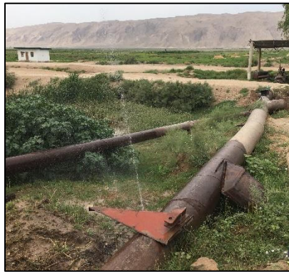
Photograph 6: Pump system drawing water from a tertiary canal to pipes that empty into intra-village watercourses in Khatlon Province, Tajikistan. The pump is operated and maintained by a local resident who took the job when no one else in the village felt qualified. Having studied physics in grade school made the transition easier, he explained, but otherwise he has learned everything related to the pump system on his own. Despite his care, leaks have sprung all along the pipes leading from the pump station into the village. A lack of funds has led to improvised solutions like red piece of metal pictured, which is successfully blocking a leak. Photos by author.
