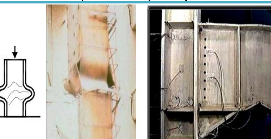
Figure 4. Damage in steel elements (CENAPRED, 2011)
