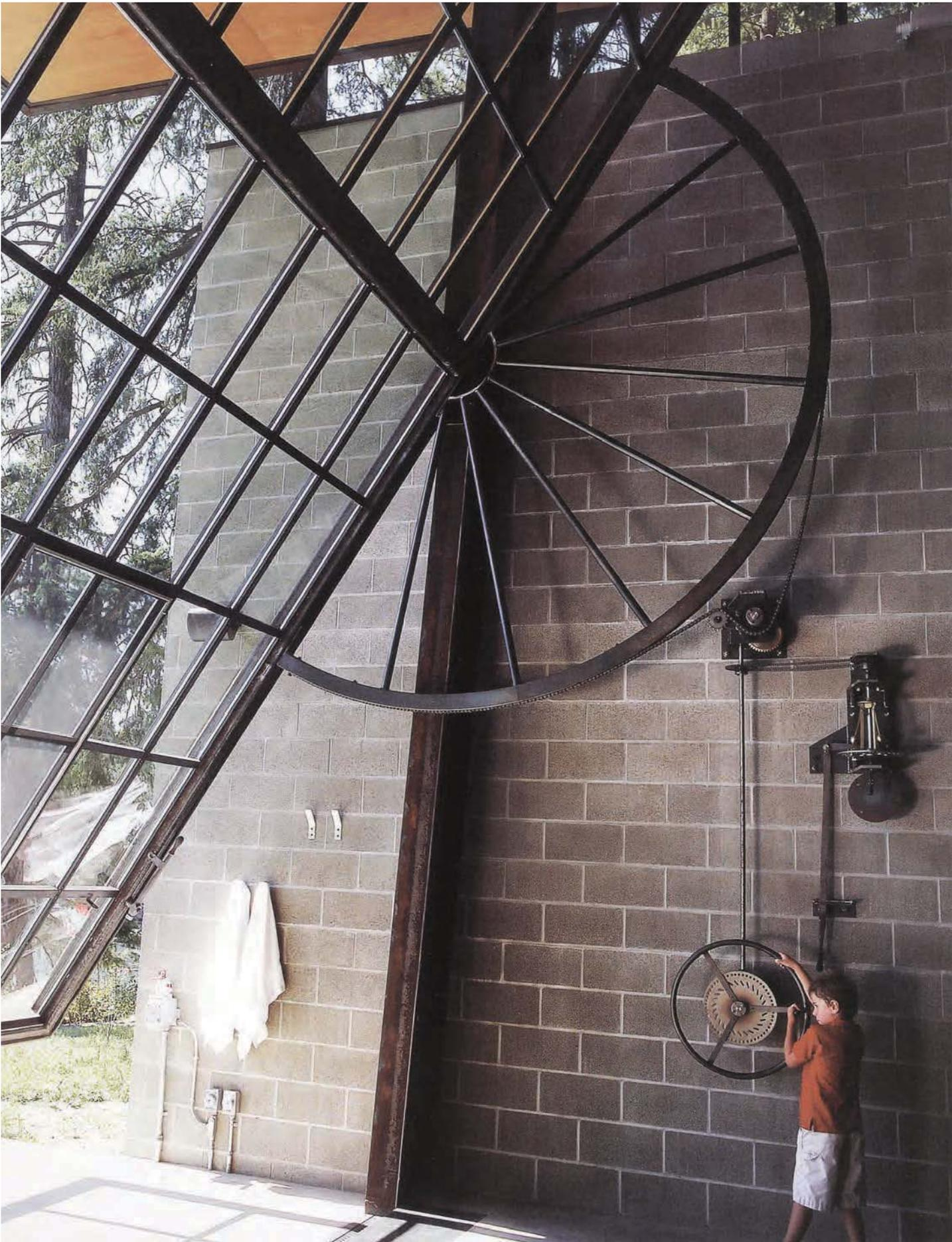
Figure 117: The gadget can be operated by the client's own son; gear ratios make this possible.
