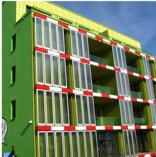
Figure 5 . Algae Building real imagery shows the algae as a clear panel, green only from the paint.
