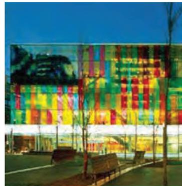
The Montreal Convention Center Expansion by Saia Barbarese Architects aims to create a vibrant public, inviting community center. The outer facade is colored glass. Behind this facade there is a walkway and then either a mirrored wall or concrete wall which give different effects. The mirrored wall almost blurs the colored structure and lighting together to look like a melting painting. The concrete takes on the color of the transmitted glass
