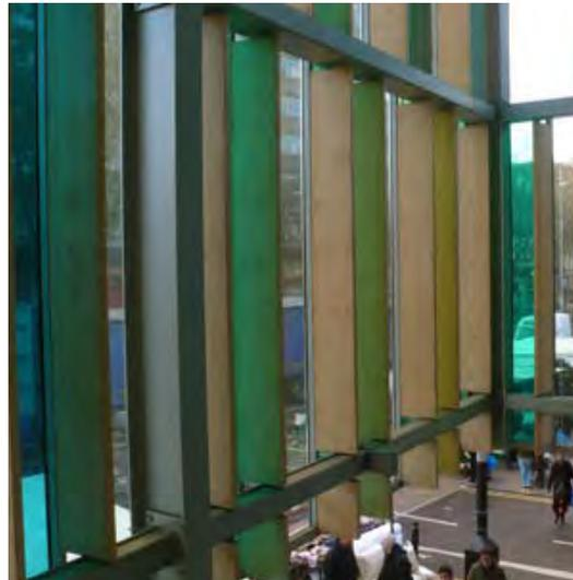
Figure 7 . The Idea Store has a combination of clear and varied color glass panels that cast green shadows on metal fins and the floor.
