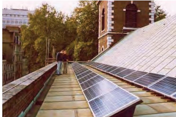
evidence of PVC from the ground. The panels were applied in a tacked on fashion on the flat part of the roof so they would be unseen. Although not the most architecturally interesting advancement, they set out to prove a historic grade building could apply PVC unnoticeably. The building adhered minimal damages to route electric wires to the church's power supply.
