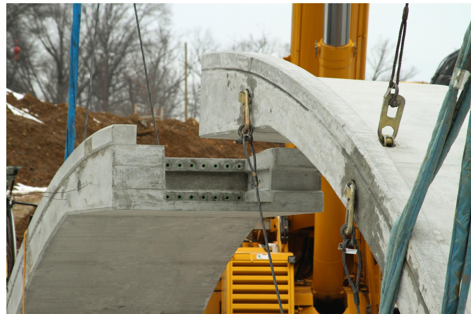
Figure 1. Precast concrete arch being placed into position. (Bloodgood, 2015).
