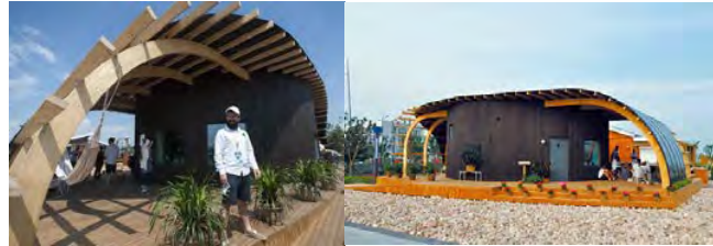
Figure.5. Curved roof of Halo
