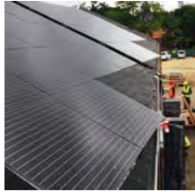
Figure.4. Slope roof of BER
