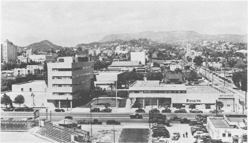
Fig. 7. Station KNX, Hollywood, California, 1936-38, William Lescaze, architect; Earl Heitschmidt, associate architect.
