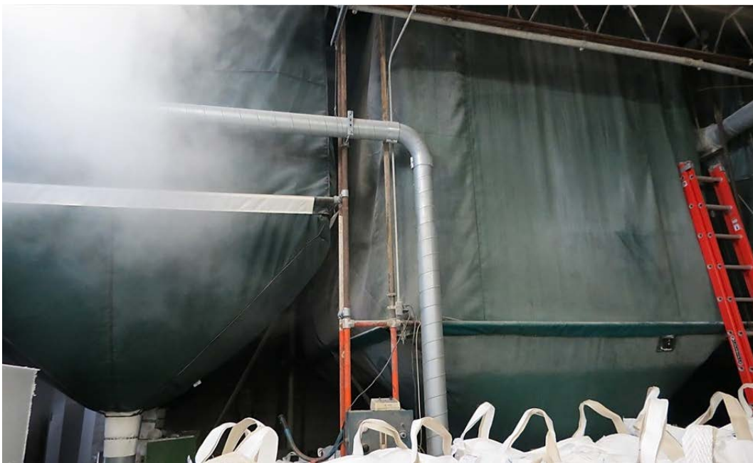
Figure 1.3 Aging silos approximately 2 X 6 X 6 m (image from field testing)
