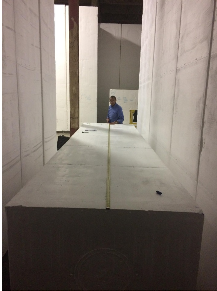
Figure 4.7 Measuring dimensions of EPS geofoam blocks
