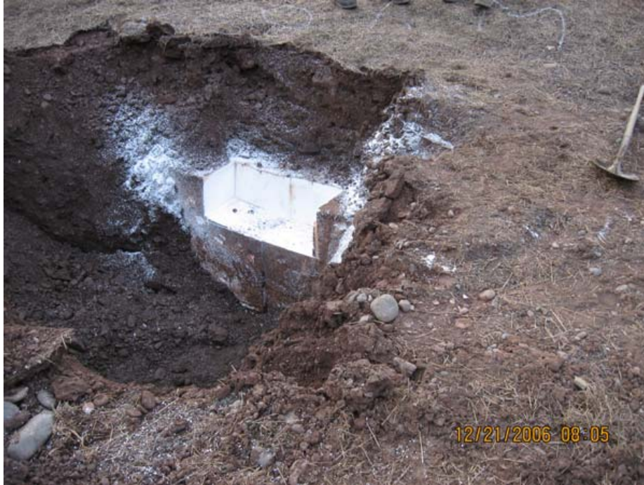
Figure 2.15 Block sampling of geofoam from a test pit along I88 (NYSDOT, 2007)
