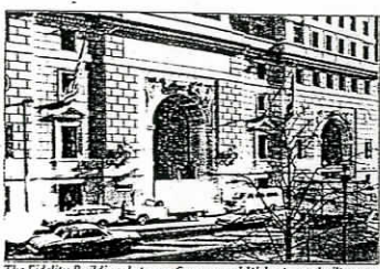
The Fidelity Building, between Sansom and Walnut, was built as one of the city's largest and most luxurious office buildings.
