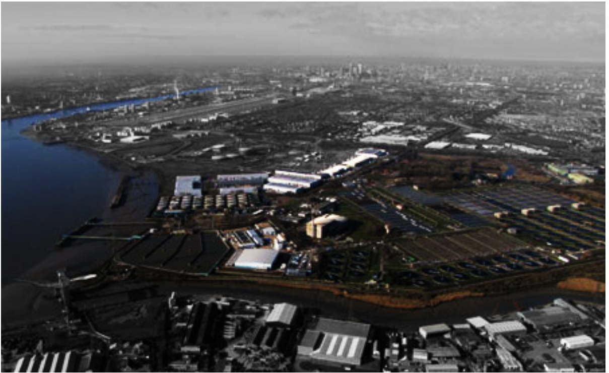
London Beckton Water Filtration Treatment Plant. The largest facility in the EU. The security is as high as a maximum security prison. Water is unloaded from France/Wales and England. This is a transnational space of water. A private infrastructural enclave mixing water from multiple geographic locations
