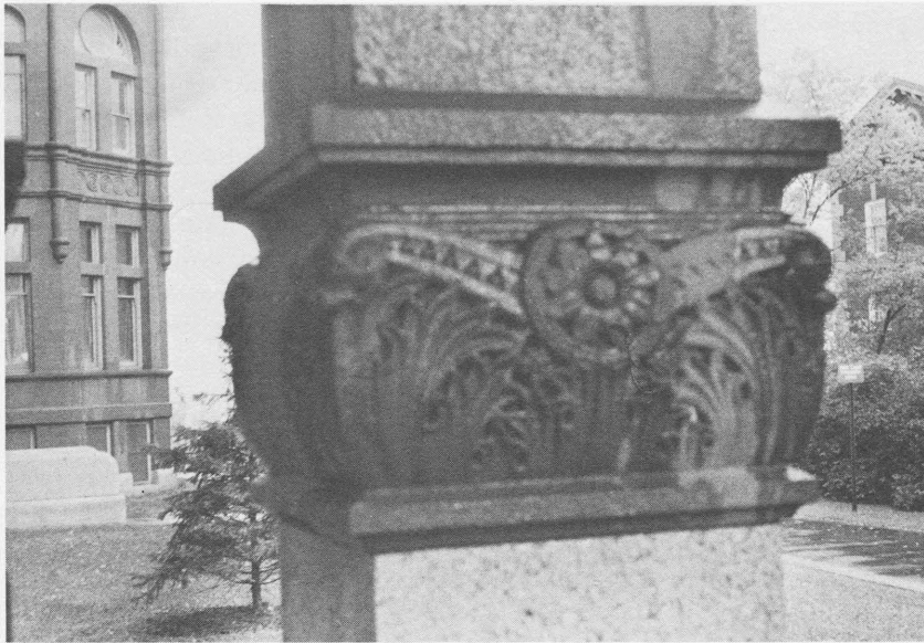
Fig. 10. Terra-cotta sunflower motif in capital, porte-cochere, east facade, Crouse Memorial College, Syracuse University, Syracuse, New York. (Photograph by E. Hardin)
