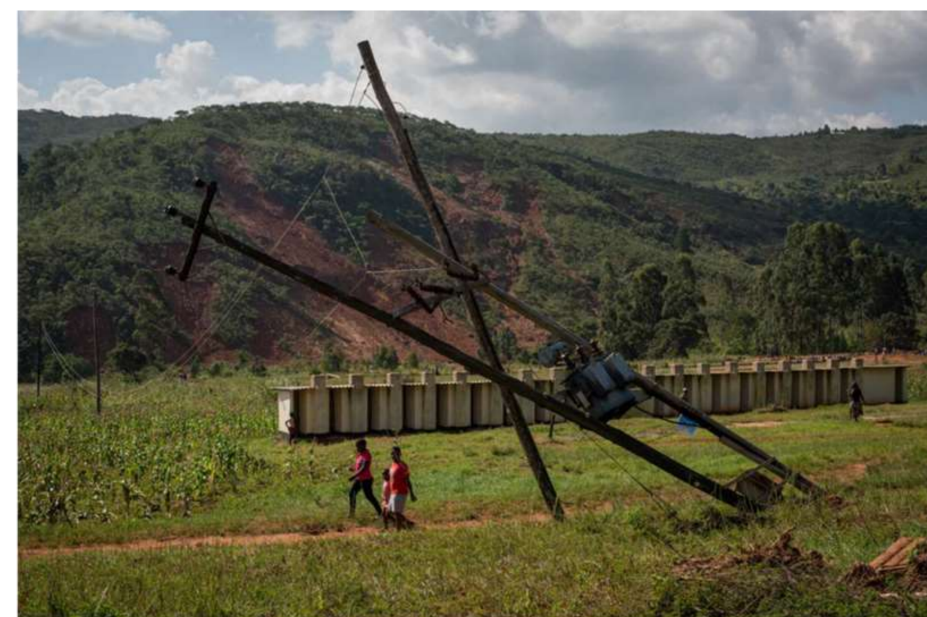
Figure 2: Environmental and infrastructural damage due to Tropical cyclone (Source: Chatiza, 2019)
