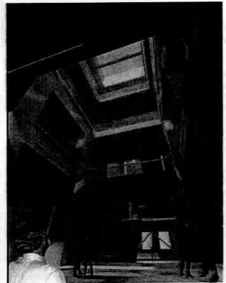
View from first floor up through replaced atrium
