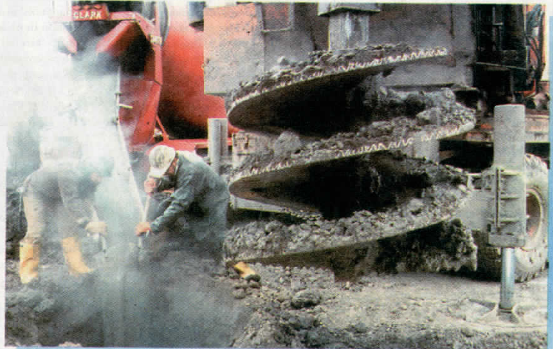
An illustration from Theodore Ceraldi's e-book, depicting caisson operations at the work site of the Institute for Human Performance, is pictured above. (Photo by Theodore Ceraldi)
