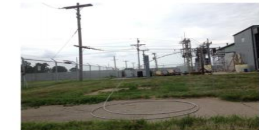
Figure 3: Downed conductor on a High Impedance Surface [2]
