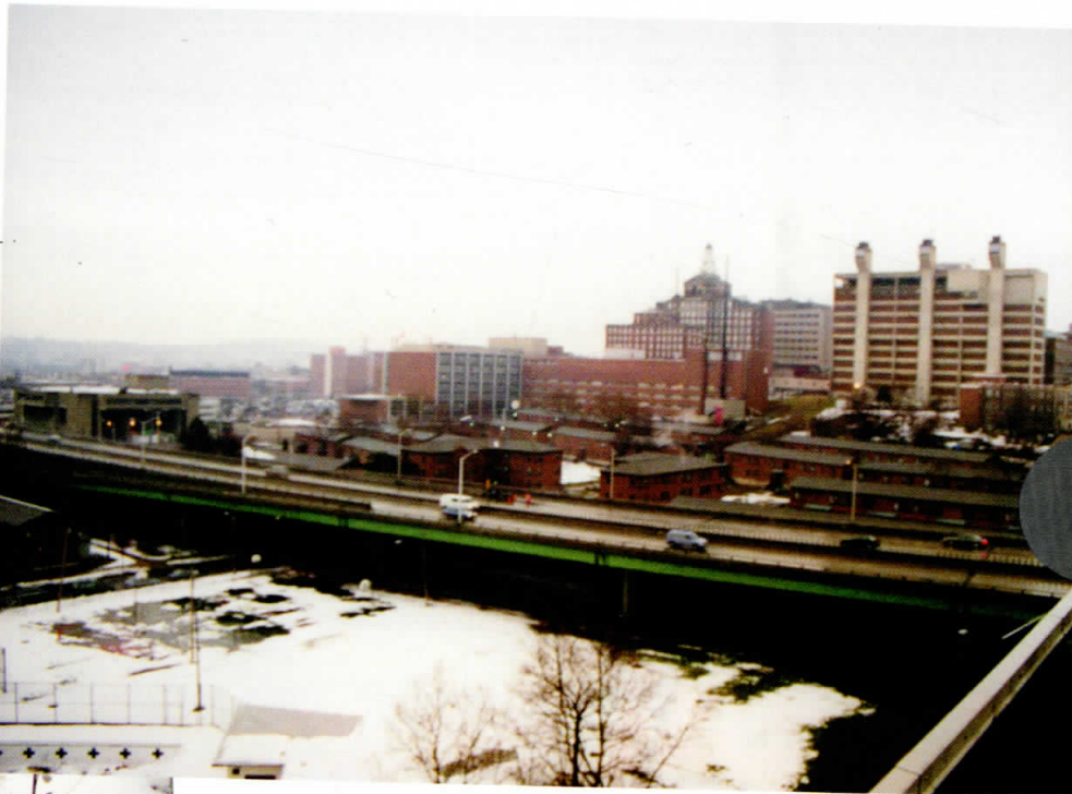
Site overview from top of Steam Station.
