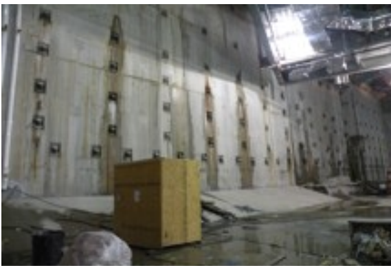
Figure 1. Reinforced concrete slurry wall. Image taken by the author from inside the halls of the 9/11 Memorial Museum while under construction, February 18, 2011.
