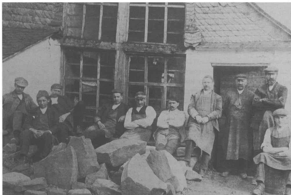
Figure 11. A group of cutters with the remains of a cutting wheel that exploded. Such an accident usually resulted in fatalities. The absence of military caps on the workers suggests that this picture was taken before World War I. The death toll on the cutters in that war was much higher than for the population in general since nearly all cutters ended up either in the infantry or the artillery.
