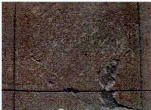
Cracked Pavers
