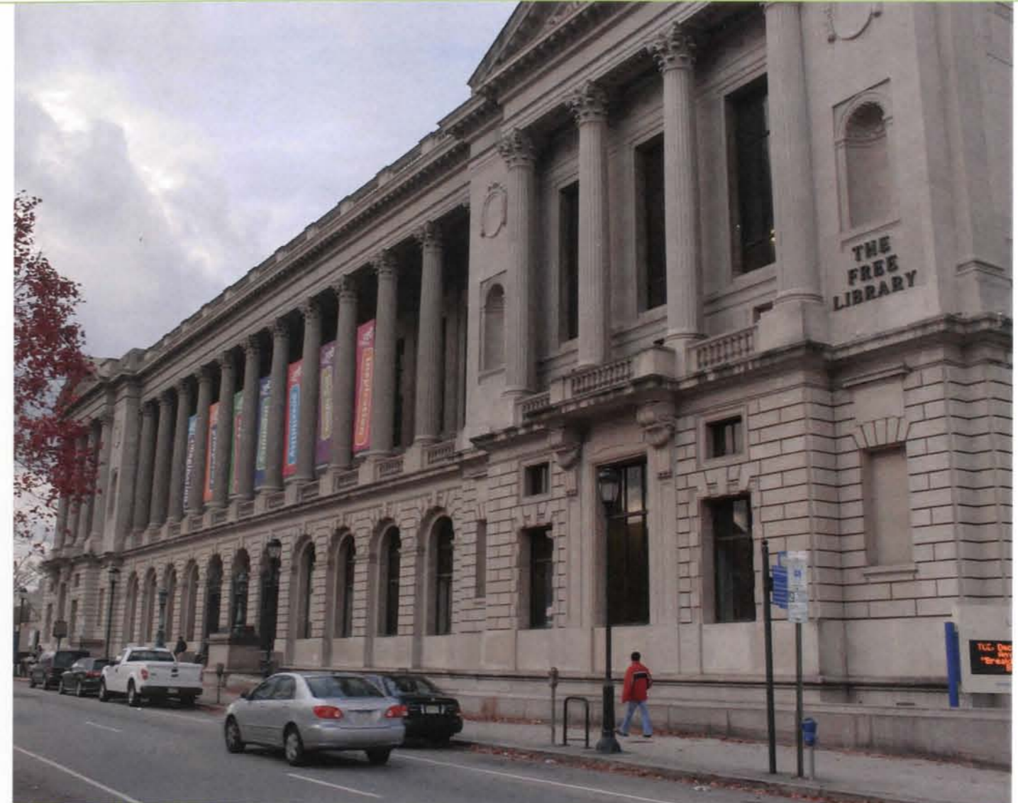
FLP Eastern (Front) Facade
