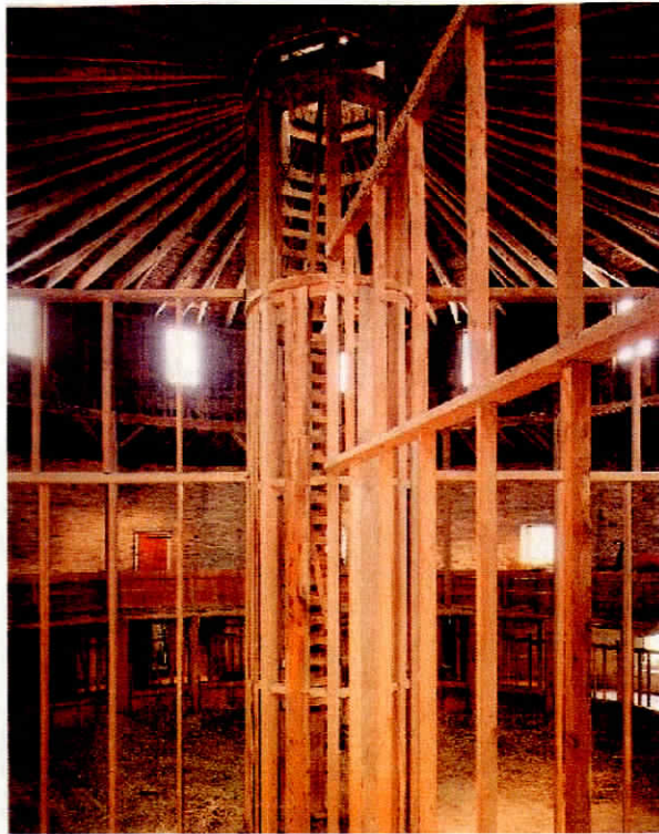
Interior of Round Barn, Hancock MA
