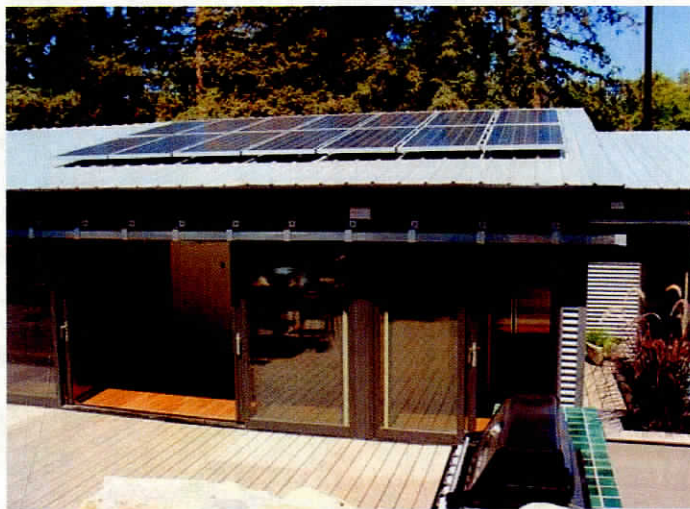
Prefab Glidehouse feature roof-mounted photovoltaic cells
