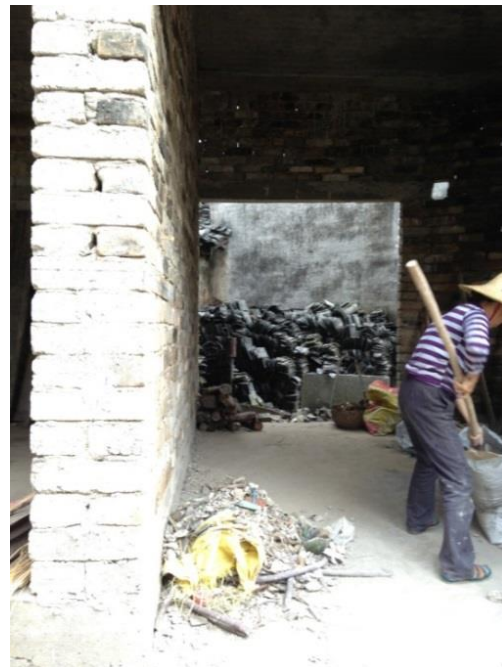
Figures 5.4–5.5 Construction of modern houses in Xucun. (By author.)
