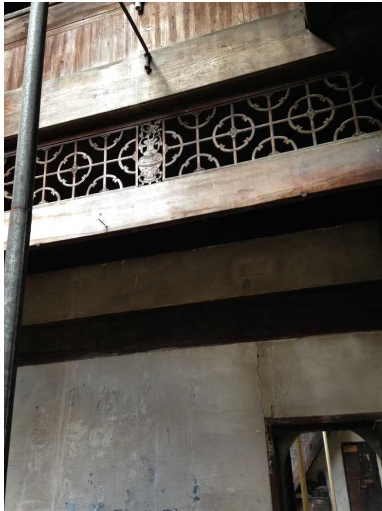
Figure 5.6: Inside a closed private house. (By author.)
