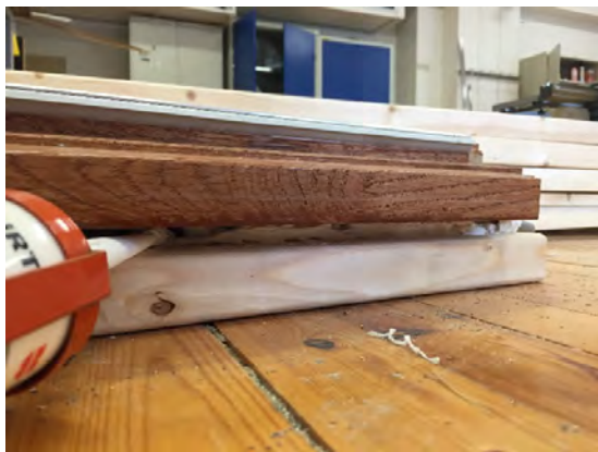
Figure 7. Application of silicon compound.
