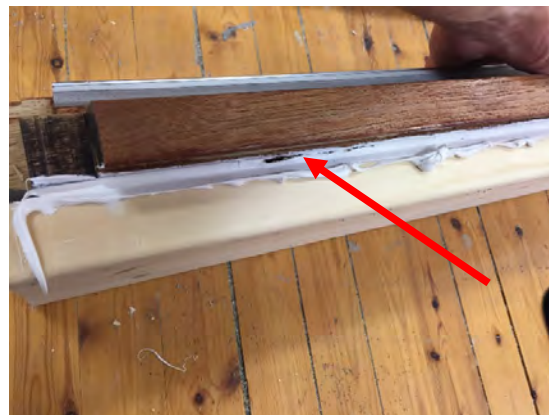
Figure 8. Small defects in the silicon compound was found by closer inspection.
