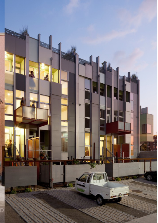
FIG 27 - Back view of project
