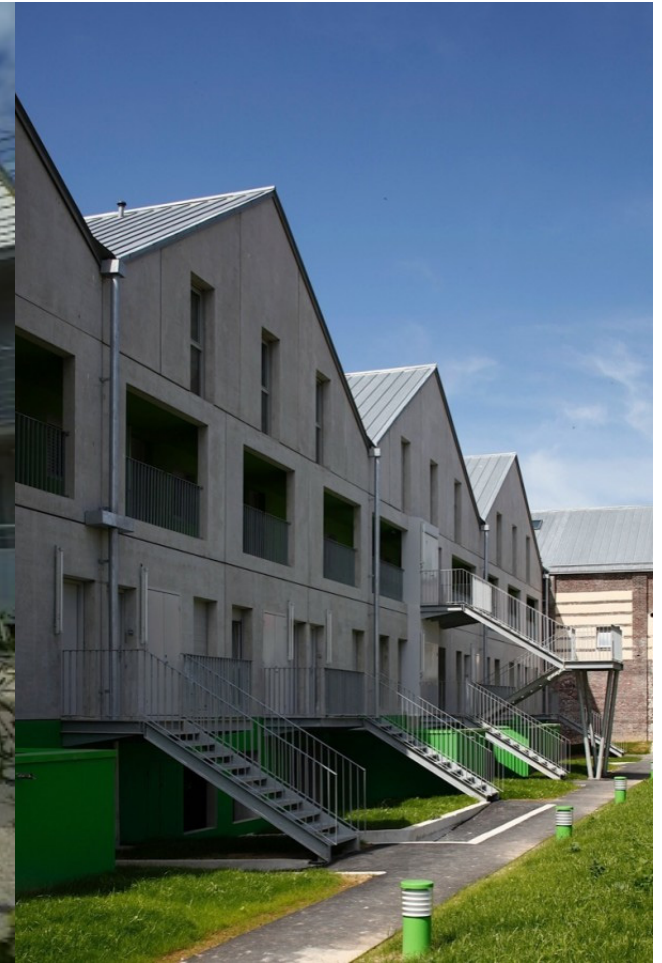
FIG 39 - View of the north elevation
