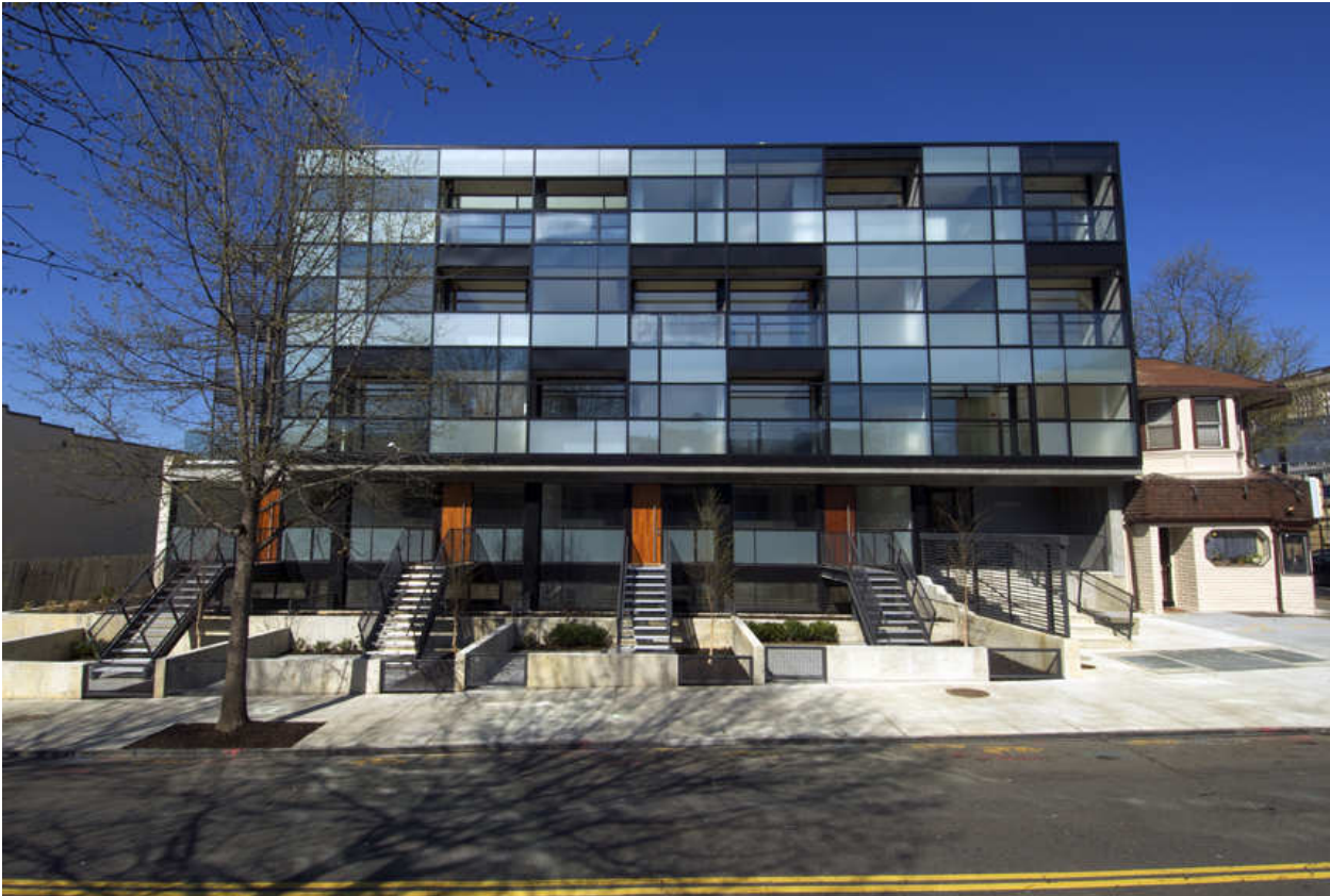
FIG 33 - Back elevation of the project showing private garden entrances to the duplexes
