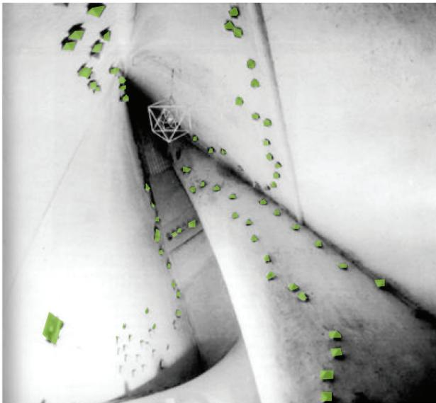
Fig 9\_ 350 speakers were installed to create the desired aural atmosphere.
