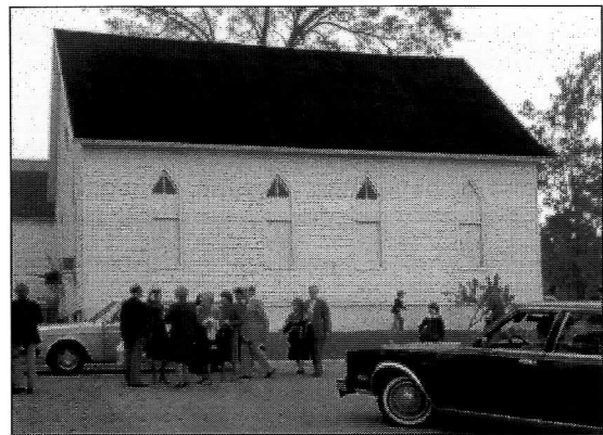
2. B’nai Abraham Synagogue, Brenham, Texas (USA), built in 1893. This was the second synagogue built by the Brenham Orthodox Community; the first one, also a wooden building, was destroyed in a fire soon after its erection. The simple wood–frame building combines elements of American vernacular church architecture with an interior organized and decorated to recall Polish–Lithuania synagogues; photo by Shirley Moskowicz Gruber.
