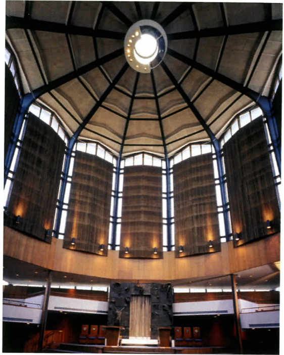
XXXVII. Temple B'rith Kodesh, Rochester, NY; Pietro Belluschi, architect (1963). Belluschi combined the Eastern European references supplied by the congregation's rabbi and his familiarity with wood learned as an architect in America's Pacific Northwest; photo by Paul Rocheleau.
