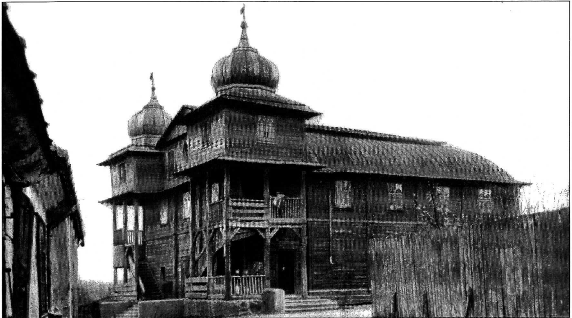
3. Synagogue, Gąbin, Poland. Two-tower façade; photo from: M. and K. Piechotka, Wooden Synagogues (Warsaw: Arkady, 1959).
