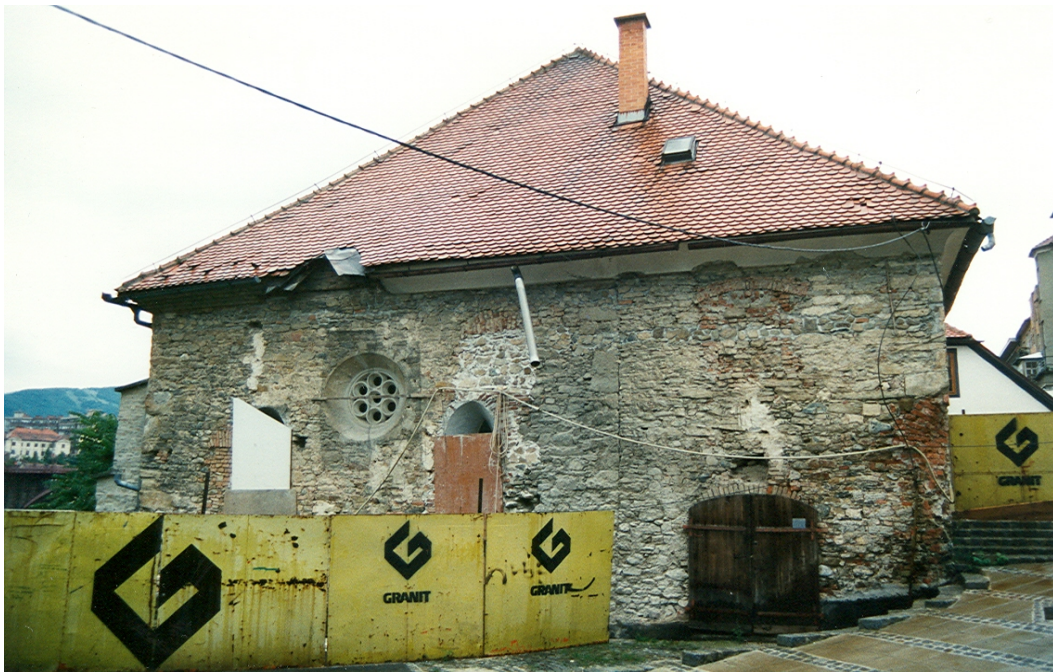
Figures 33, 34. Maribor. The synagogue, sited in the former Jewish quarter next to the town's defensive walls and turned into a church by the year 1501. In recent years, excavation and restoration of the building has attempted to recover the original form of the synagogue and to restore its medieval appearance. Top: North façade. Bottom: East façade.
