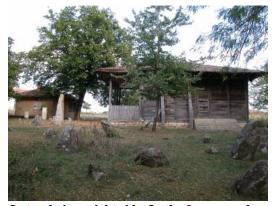
Lateral view, right side. In the foreground, the remains of the cemetery. At the far left, the former *mehteb*. Note the older wooden buttressing of the wall of mosque and more recent brick and concrete reinforcement at the base of the wall.
