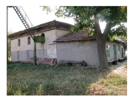
Oblique view from left. Note bricked-in portico, improvised access to minaret, cracks and buckling at left front corner, and laying of brick in an attempt to shore up wall.
