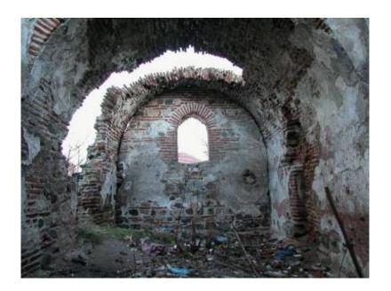
Interior. The sanctuary. Note the partially collapsed state of the barrel-vault and the buckling of what remains of the left-hand side of the vault at its juncture with the *mihrab* wall.
