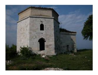
Lateral view of southern side of monument from the summit on which it is set. Note the fine quality and precision workmanship of the marble facing. Some cracks and missing pieces are evident but, otherwise, the exterior walls have survived the centuries well. The tambour atop the marble walls is made of rubble coated with plaster, a technique that helps us date the monument to the 15<sup>th</sup> century. The tambour was renewed during the restoration of the monument during the late 1960s.
