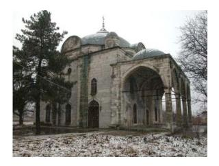
Oblique view from side. Note the doorway cut into right-most of the three ground-level windows on the left of the building. Also note apparent vulnerability to seepage of buttressing piers on lateral wall.
