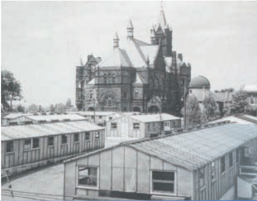
Prefabricated temporary buildings lined the Quad behind Crouse College in the years following World War II to serve as classrooms for the nearly 10,000 returning veterans that came to campus.
